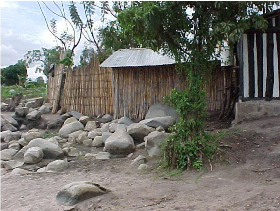
Plate 10. A toilet behind a tea house , with an open channel emptying directly into the lake
