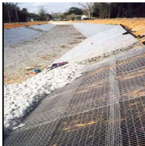
Figure 24: Rectangular wire boxes / baskets are filled with small-sized stones and used to control soil erosion on unstable banks.
