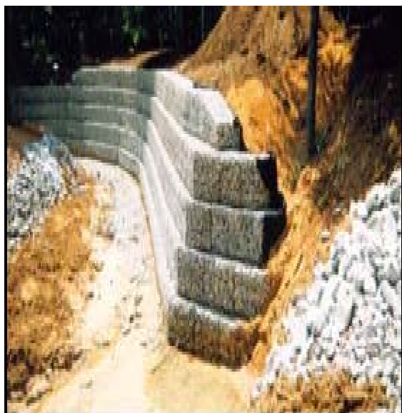
Figure 24: Rectangular wire boxes / baskets are filled with small-sized stones and used to control soil erosion on unstable banks.
