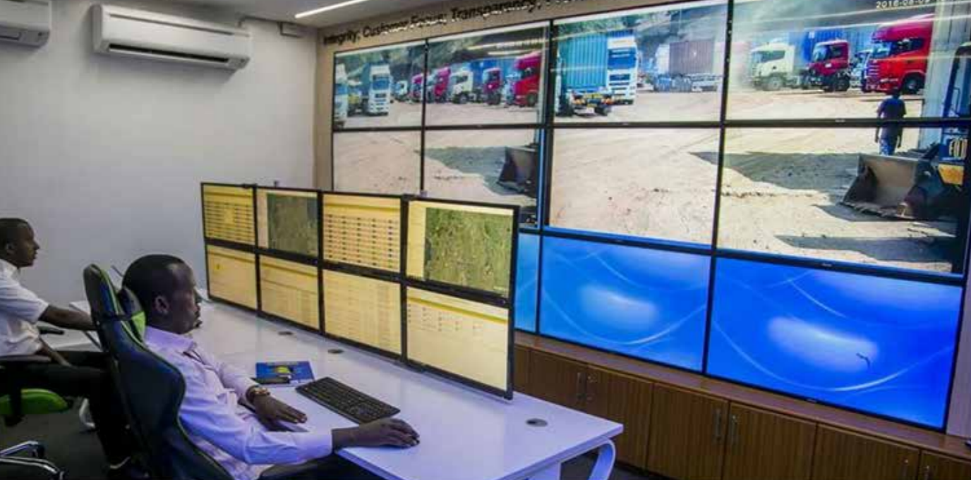
Electronic Cargo Tracking System station in Kigali, Rwanda. (Source: Photo taken by RRA officers)
