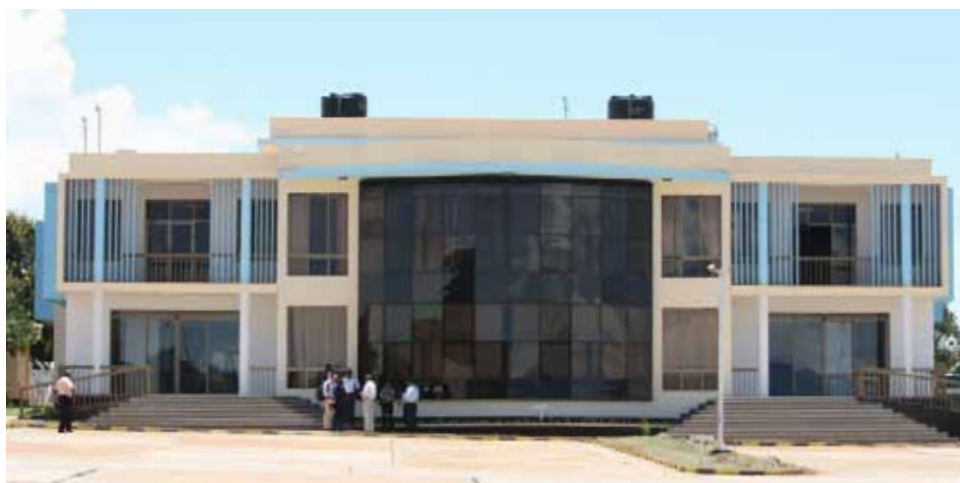
OSBP Building now ready for use at the Holili border crossing.
