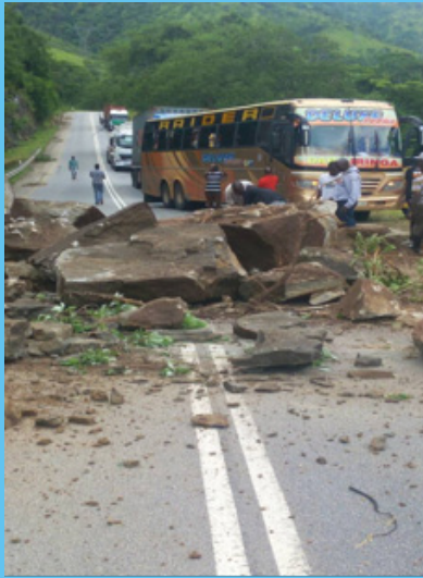
LANDSLIDE Iringa, Tanzania | 2017
