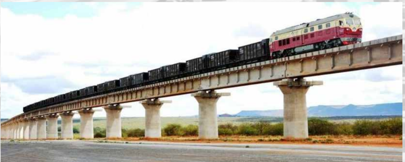
A section of the Kenya Standard Gauge Railway at Tsavo bridge
