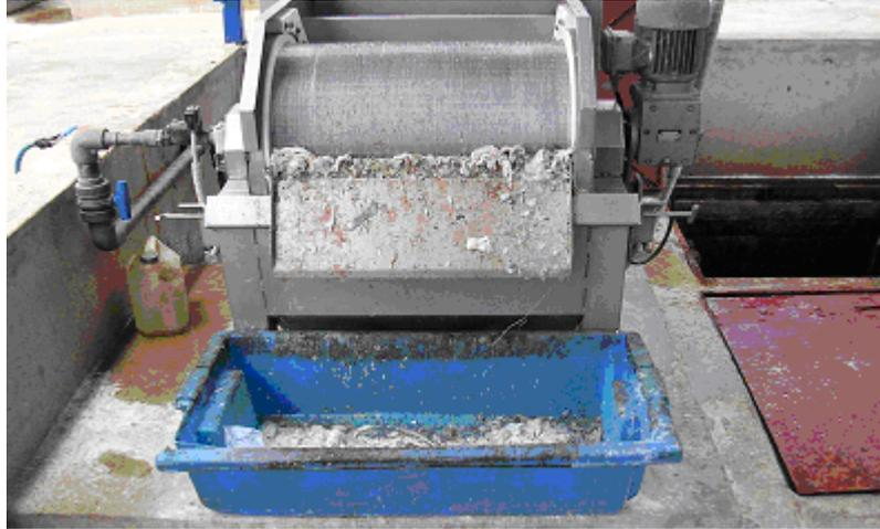
**Fig.1 Screens at Prime Catch Ltd. (MUSOMA) Wastewater Treatment Facility**
