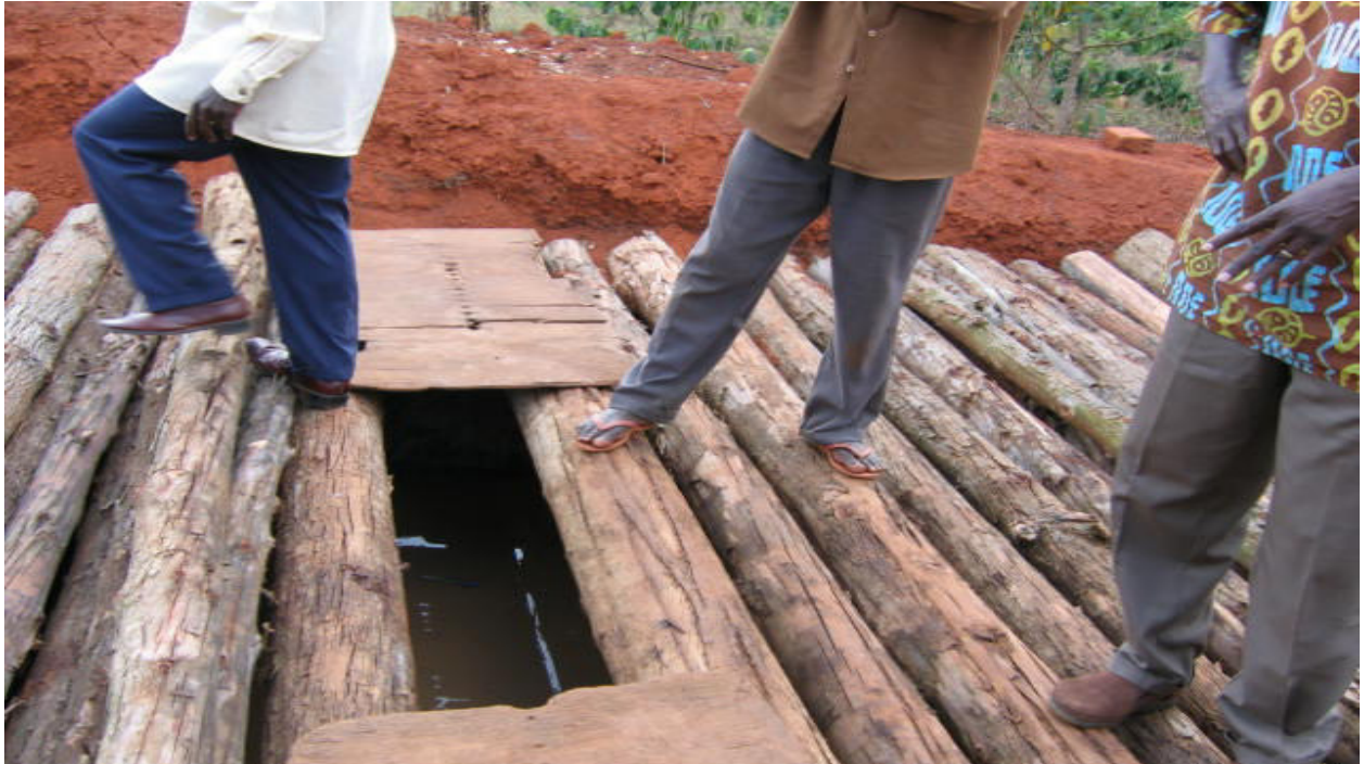
Construction of underground water reservoir
