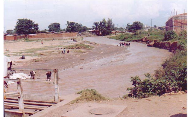
h. Threats of flood on the dwellings of the Buyenzi district in the major bed of Ntangwa River
